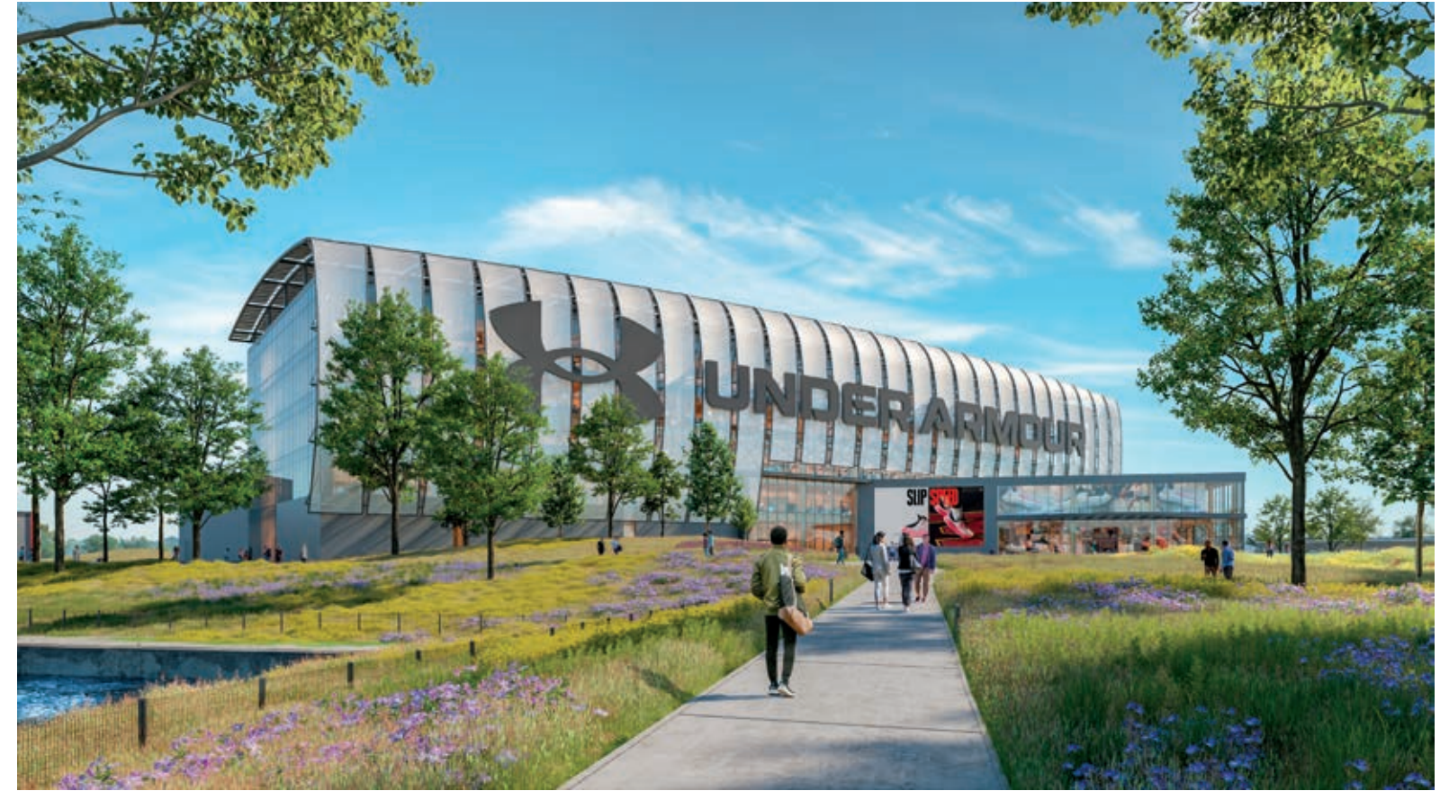
Under Armour Global Headquarters, Baltimore Net zero energy
